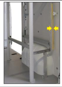
Level the block and mounting parts so that all connections are free of tension and the block is perpendicular to the floor.
